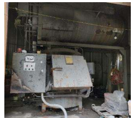
Figure 8: Example of an incinerator in disrepair
