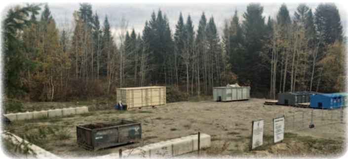
EFN's new transfer station features a solar powered bear fence and containers for (clockwise from left) large metals, household hazardous waste, bulky waste, and household waste & recycling.
